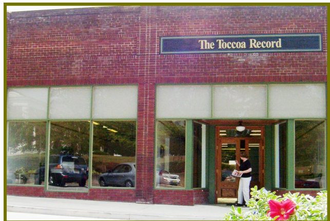
The Toccoa Record after façade renovations were complete.
